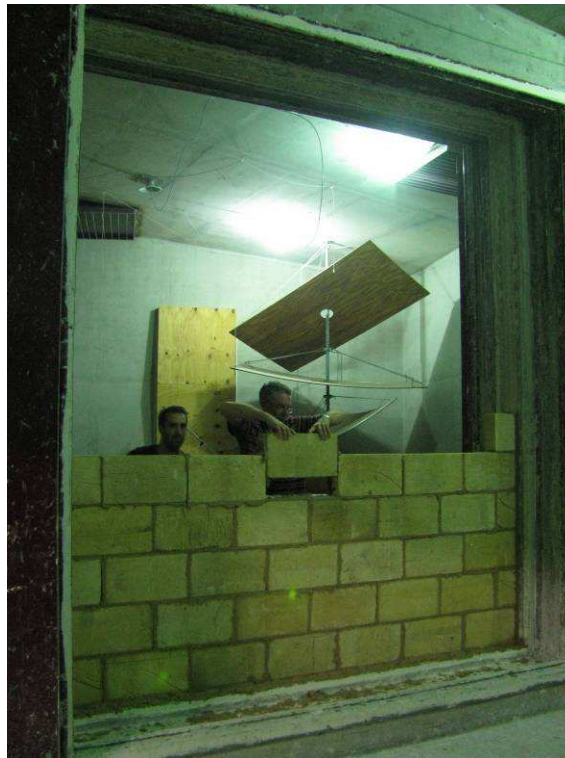
Figure 1. Construction of Timbercrete "Ancient Stone" brick wall in the aperture
